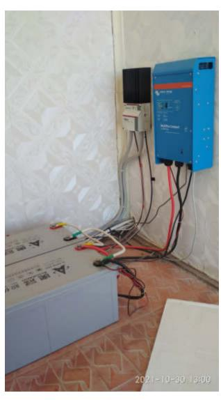
replaced the batteries for uninterruptible power supply of the entire complex of equipment
